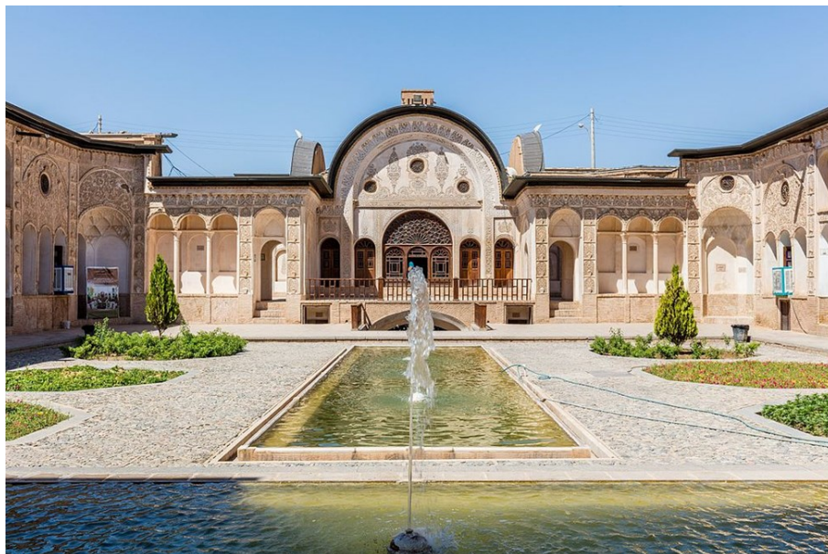
Figure 7. Tabātabāei house - Kashan
