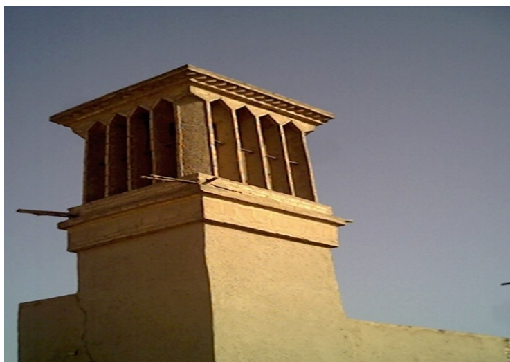
Figure 6. Wind-tower in Yazd to use wind energy as a cooling system
